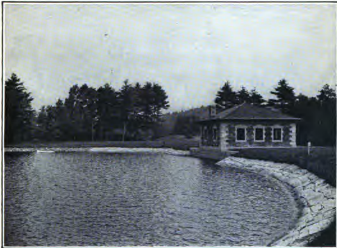
SCREEN CHAMBER, WESTON RESERVOIR
